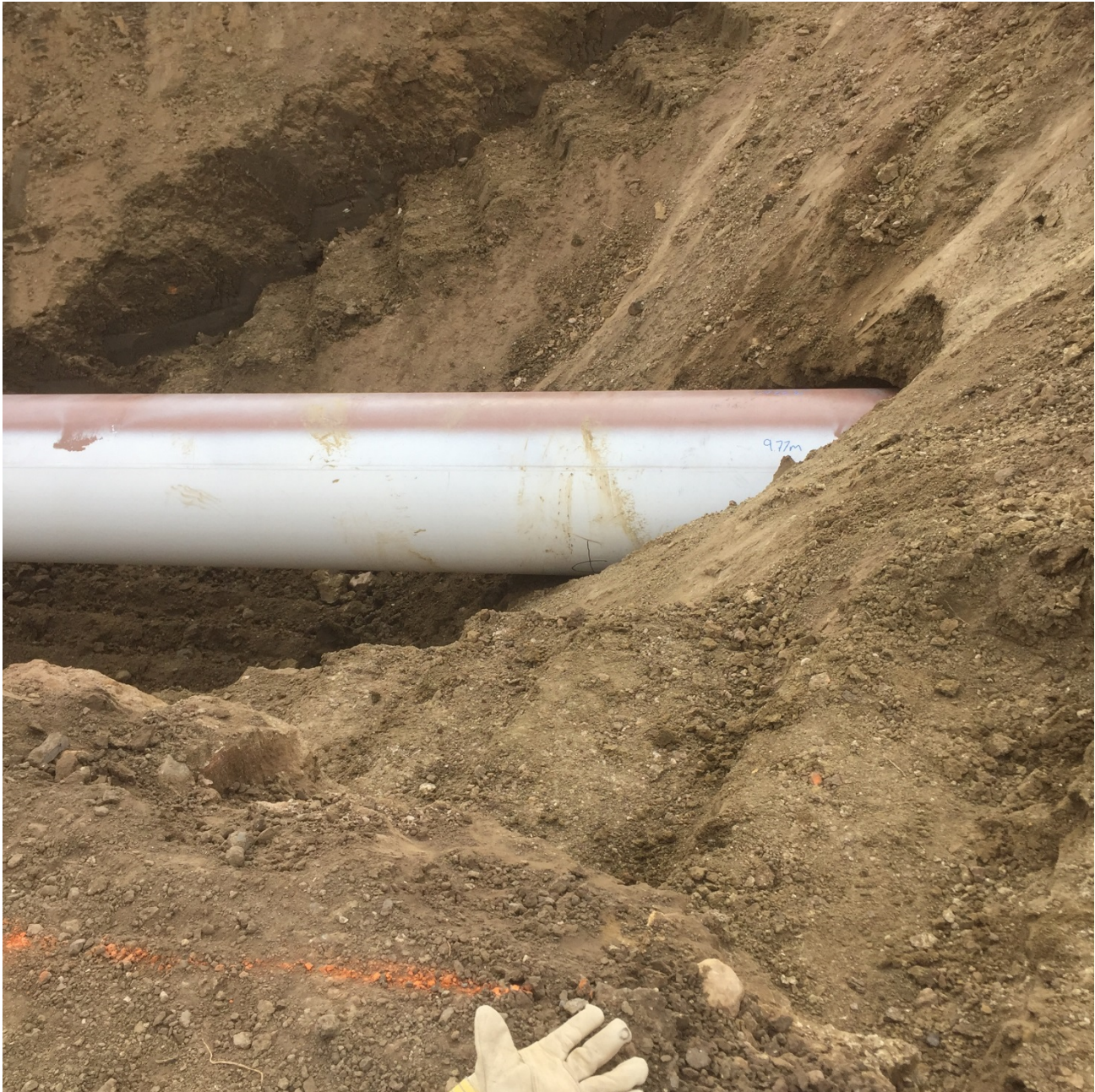
PIPELINE ENTERING BORE HOLE
