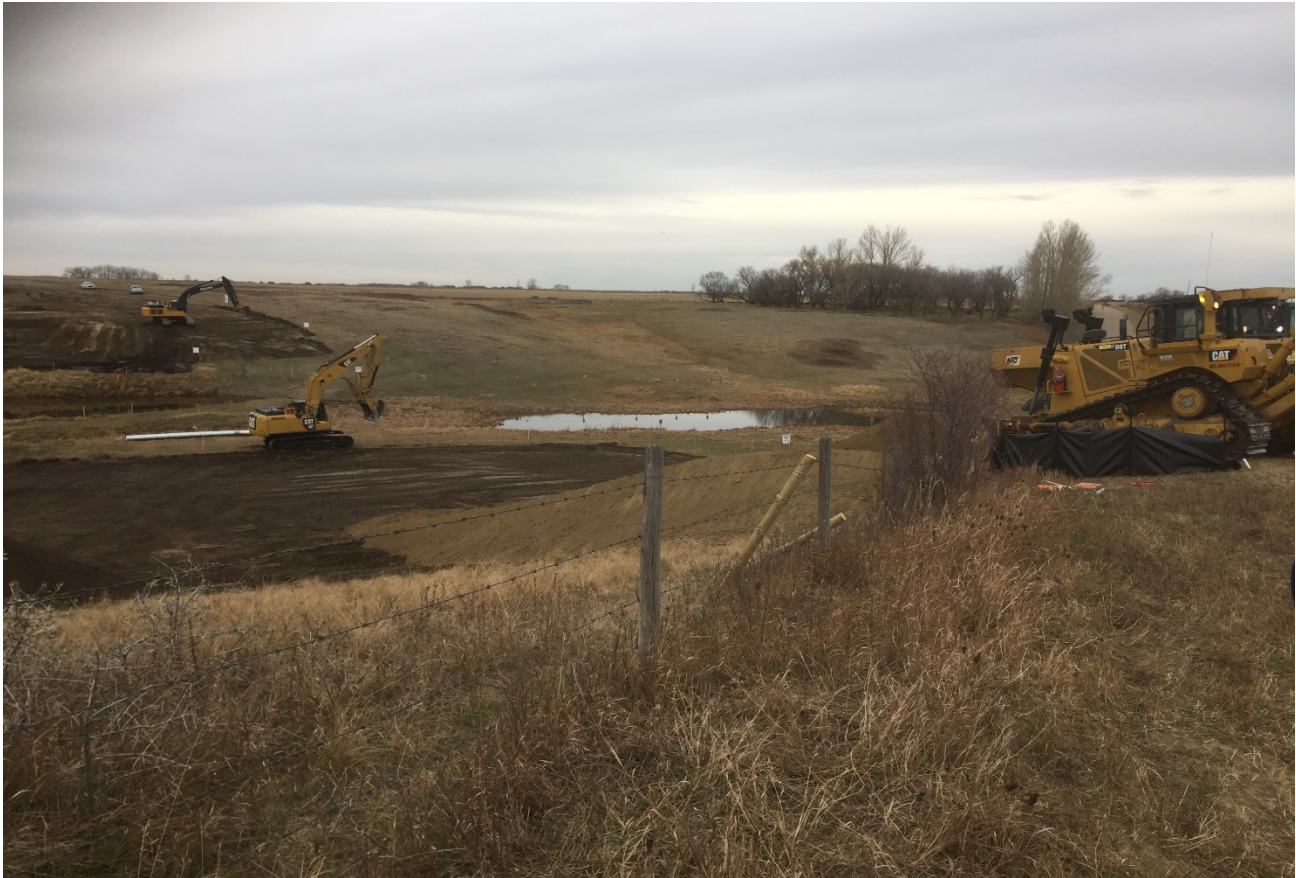
BACKHOES STRIPPING TOP SOIL
